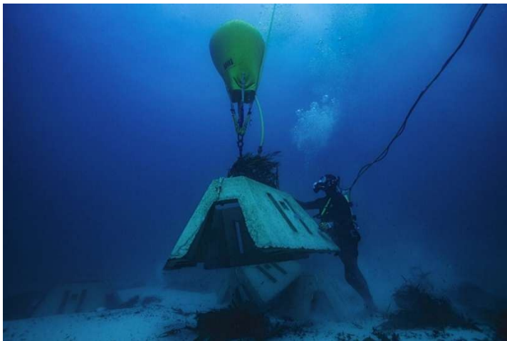
Fig. 8 Introduction of the artificial reef "Abitat" keeps the released young abalones from the hatchery in place until harvest two years later (Flinders Bay, Australia) ( A World First - Ocean Ranching - Rare Foods Australia )
