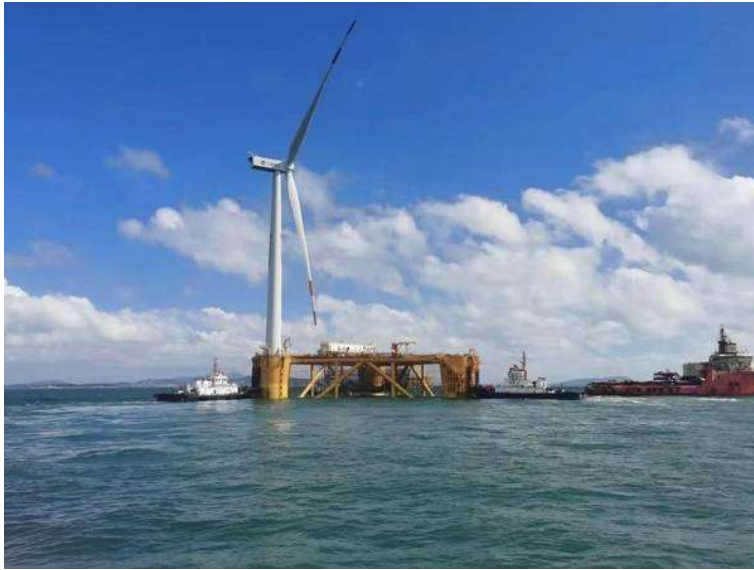
Fig. 4 Energy platform with integrated fish cage, designed by Longyuan Power Group and Shanghai Electric Wind Power Group (China) ( https://renewablesnow.com/news/longyuan-completes-maritime-floating-wind-plus-solar-project-in-china-838787/ )
