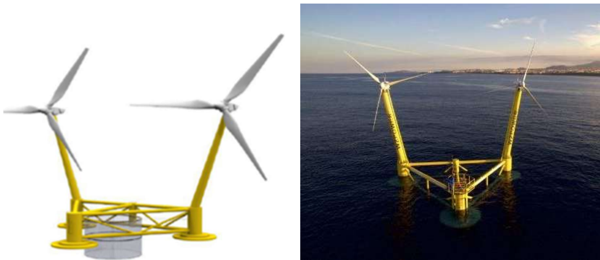
Fig. 6 Left: Design of the W2Power floating energy platform with the fish cage in the centre; Right: The W2Power energy platform at the coast of the Canary Islands ( https://cinea.ec.europa.eu/featured-projects/aquawind-innovative-multi-use-prototype-combining-offshore-renewable-energy-and-aquaculture-atlantic_en ).
